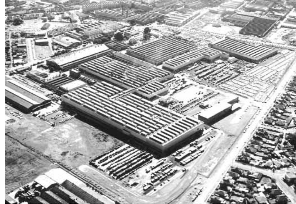
Aerial view of the Zetland site. The CAB 3 building is at the top right of the photo, with the MGB assembly line beneath the darker roof.
