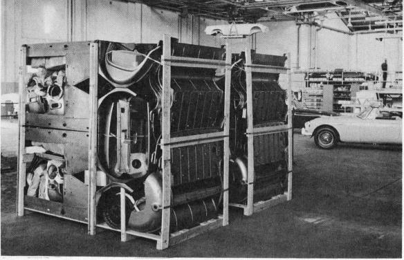
Two crates of (Midget) parts awaiting unpacking. Maximum use is made of the available space. Each crate is sufficiently large to contain almost all the parts for one car. The elevated B shell in background has just returned from paint shop, is about to be lowered on to final assembly line.
